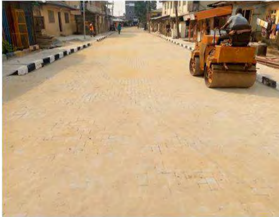
The newly constructed Akinyemi Thompson Street
